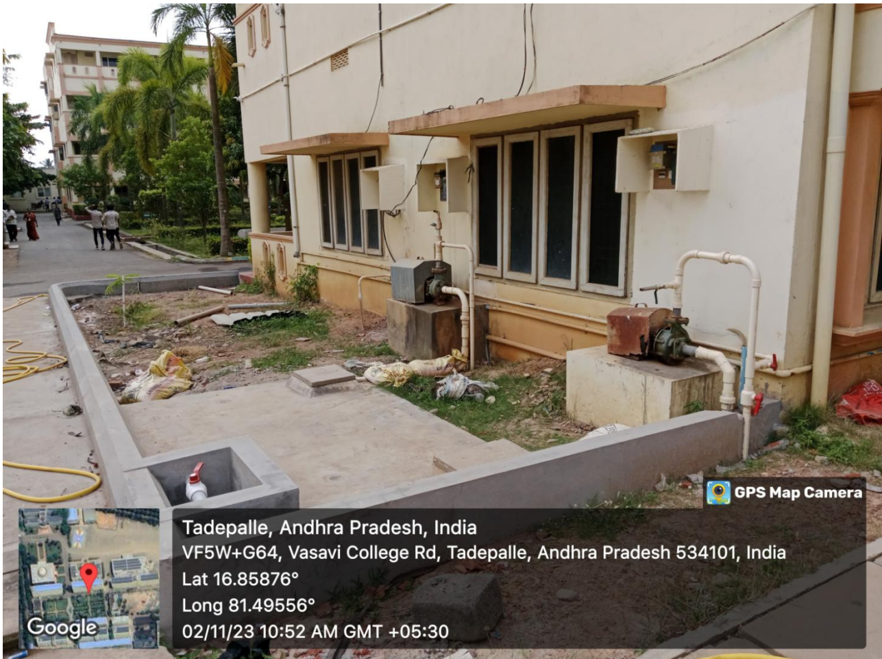
Fig. The sump with two 3HP motors near Diploma block is used to supply (Bore water) to Auditorium block, BSH block and CRC-1 Blocks wash areas.
