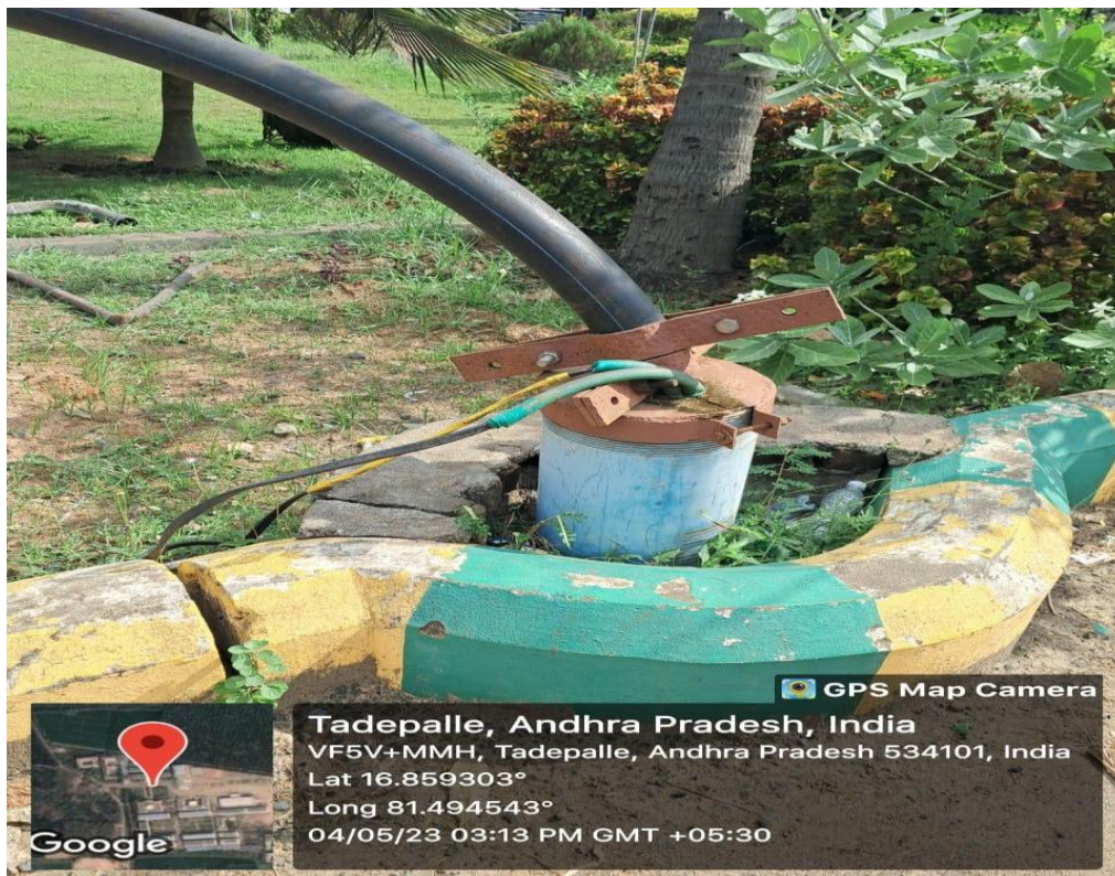
Fig. The sump with two 3HP motors near Diploma block is used to supply (Bore water) to Auditorium block, BSH block and CRC-1 Blocks wash areas.
