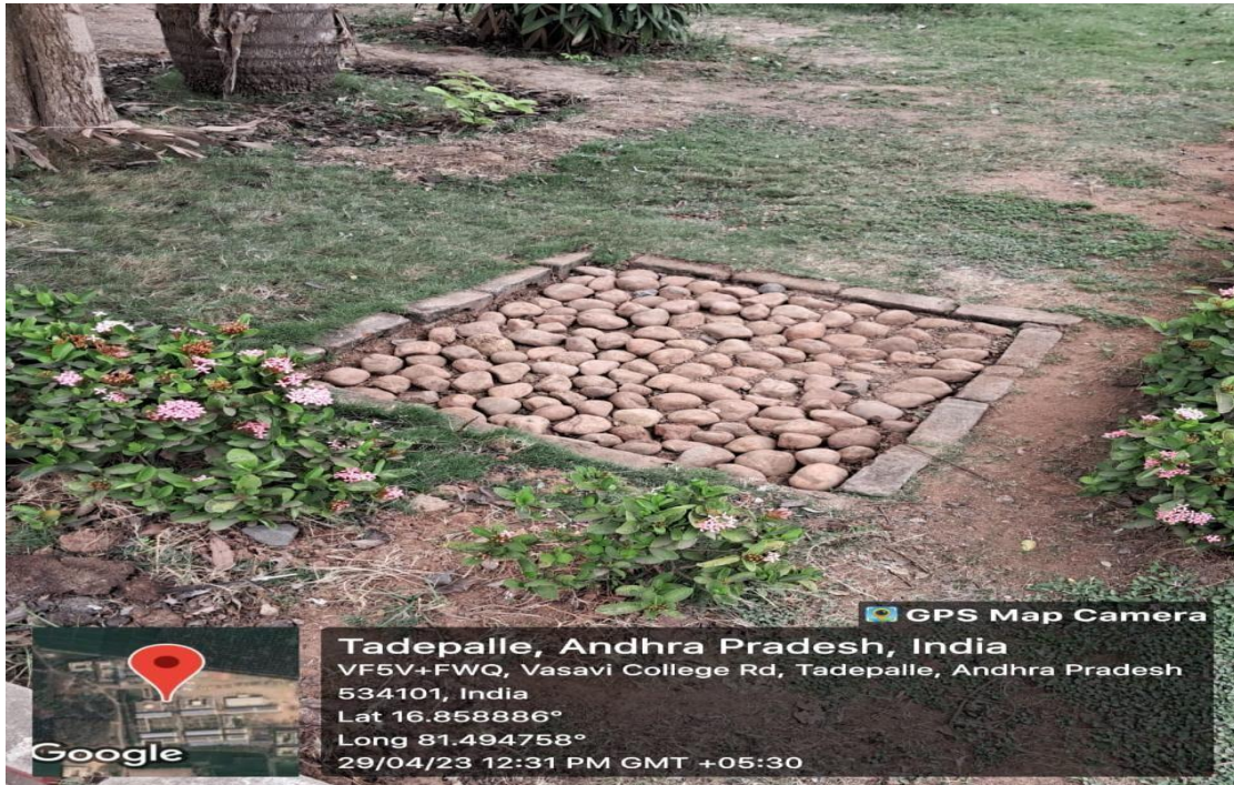
Fig. Borewell/Ground water recharging through Rain water harvesting-Pit -1 (near Main office)
