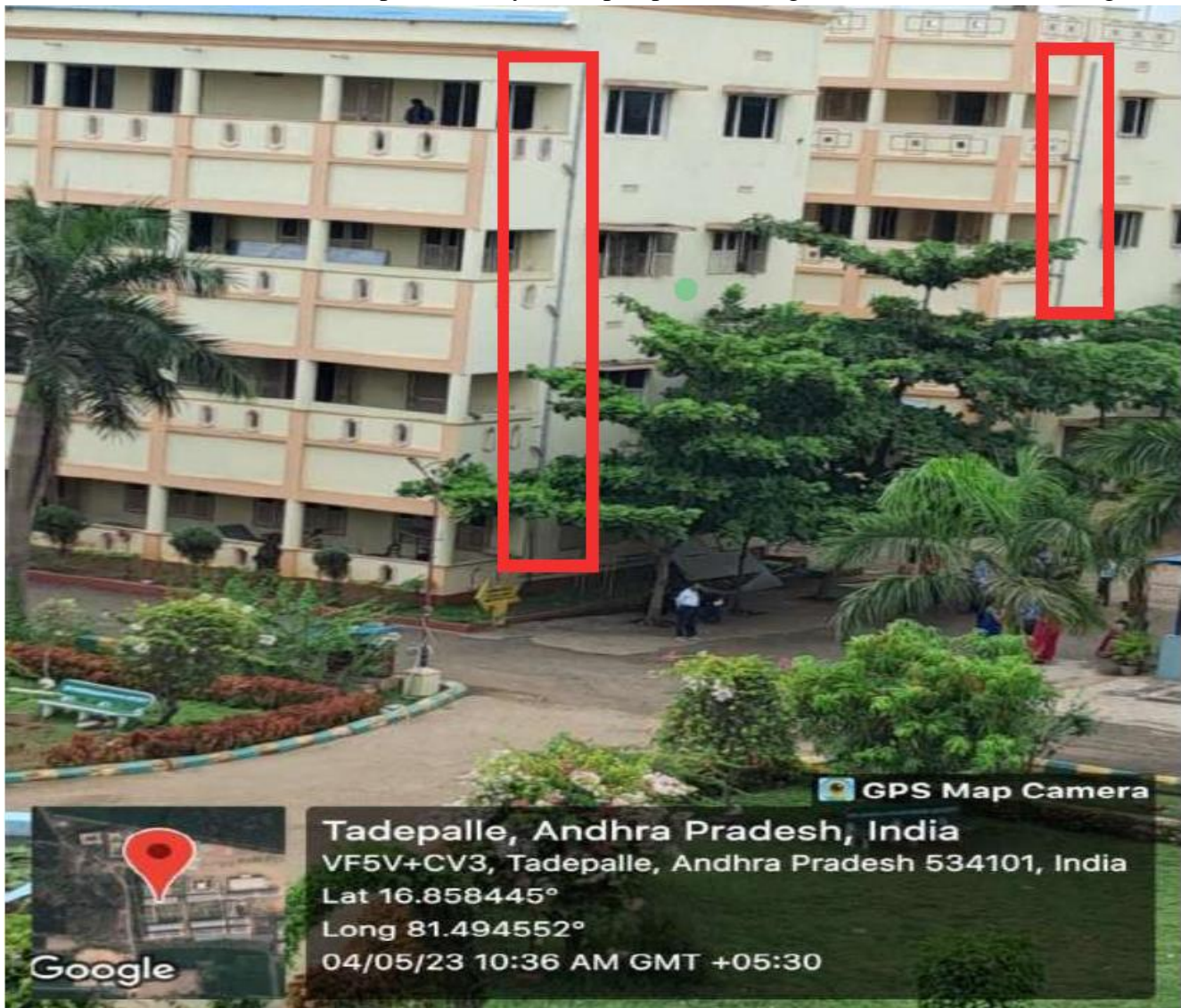
Fig. Rain water collection from roof top
